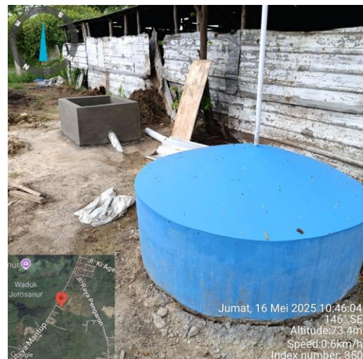
Gambar 3. Finishing Digester Biogas
